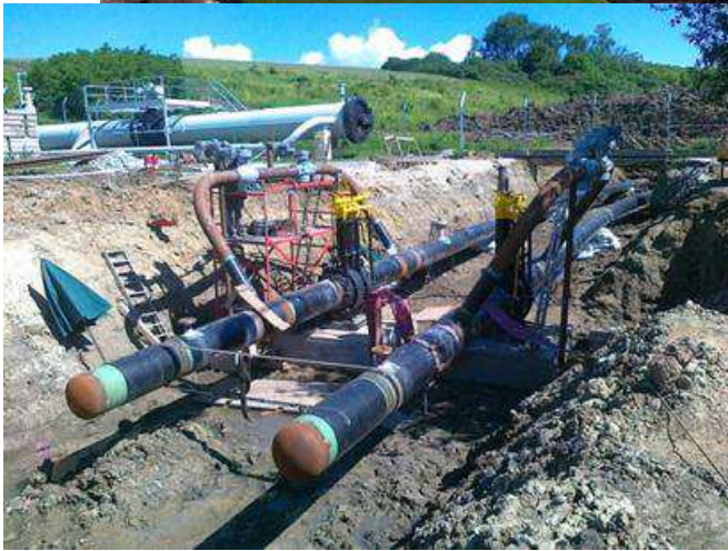
Interconnection with the existing pipe yard at CS Veľké Zlievce
